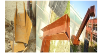
Fig 2 :- A View of Inclined part
